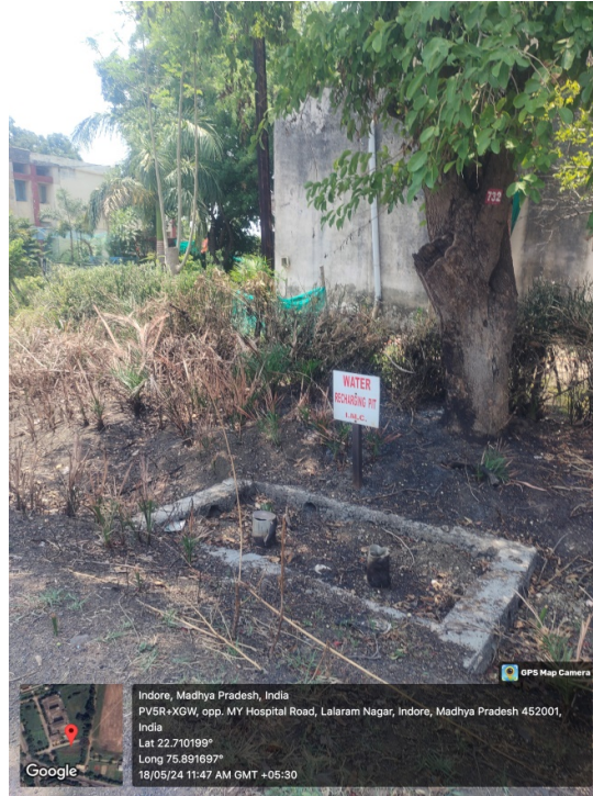
Rain water harvesting pit
