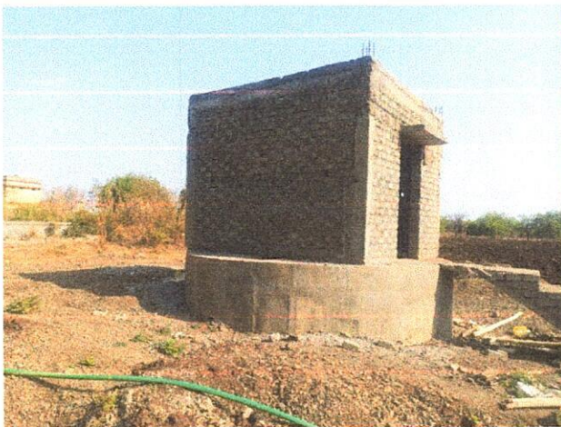
Establishment of sump well for water storage
