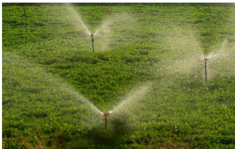
Sprinkler system for lawn watering
