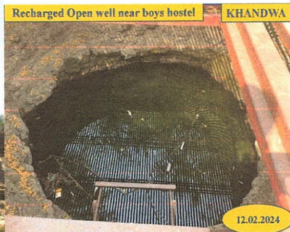
Recharged open well near boys hostel
